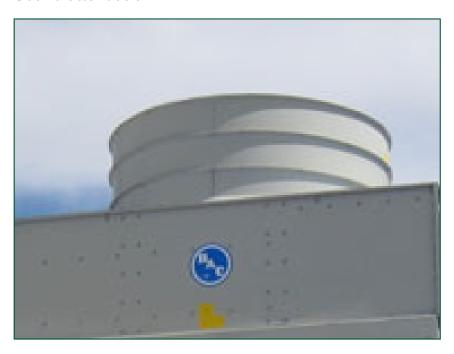
PCE condensers use **quiet and low kW axial fans**, but to reduce noise even further, you can extend your PCE condenser with <u>sound attenuation</u>:
