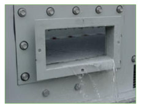
A factory-installed clean out port
