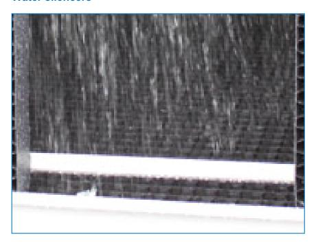
Water silencers in the basin **reduce the noise** of the water falling into the basin. They are easily removable in **modules** for basin inspection or cleaning.
