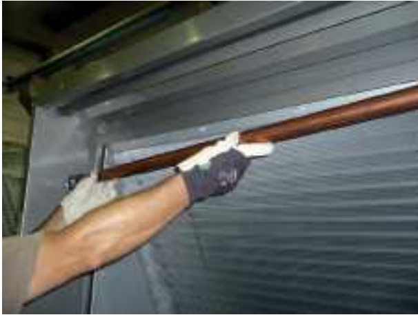
Remove copper waterfeed pipe
