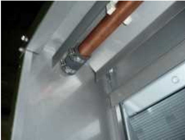
Flexible sleeve connection with sleeve clamps
