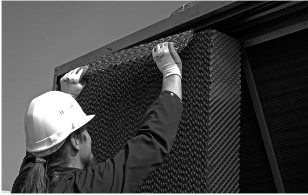
Removal water distribution pads
