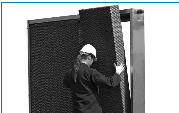
Removal of pre-cooler media
