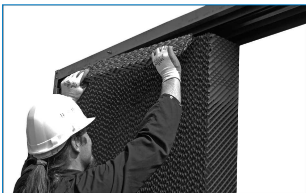
Removal of green water distribution pads
