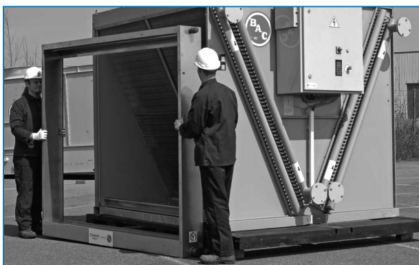
Installation of empty pre-cooler frame at dry unit.
