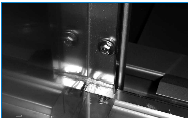
Stainless steel bolts and nuts connecting pre-cooler frame to dry unit flanges.
